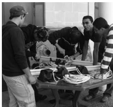
Carrying out electrical works
