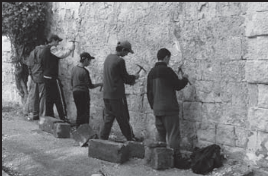
The students cleaning the garden walls from various plasters
