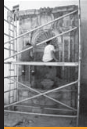
Two MCAST students during the cleaning process and discovery of the various lime washes
