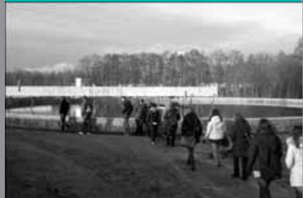
The Water Treatment Plant at Scheemda
