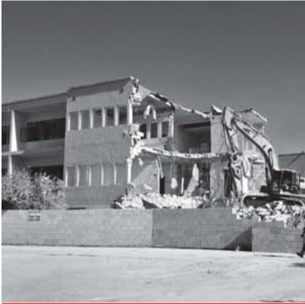
Demolishing of Institute of Business and Commerce (Block B)
