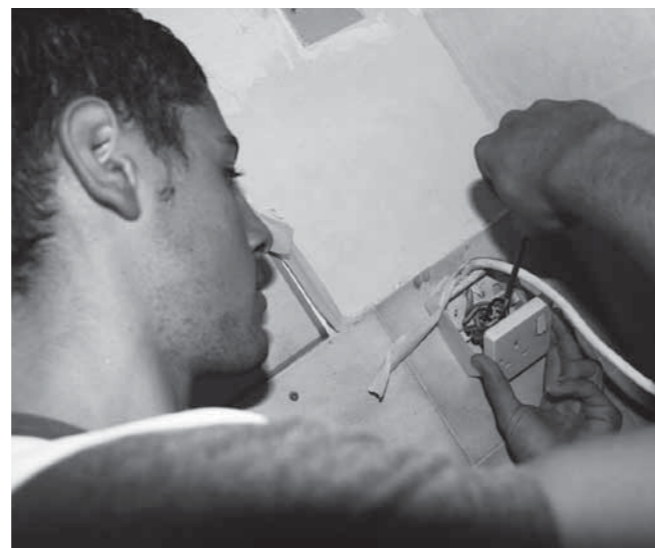
Pawlu Portelli carrying out electrical installation work at the Centre
